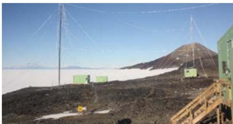
The Scott Base. ionosonde mast (left) and winds radar mast (right).
