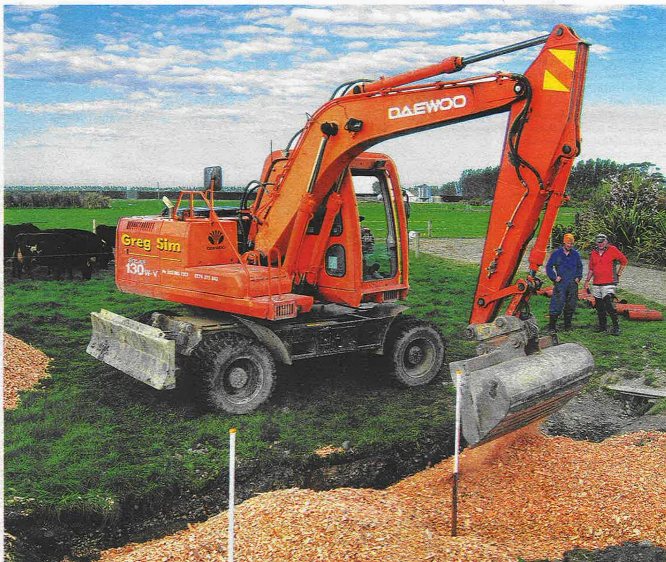
The building of a 30m<sup>3</sup> woodchip bioreactor constructed to intercept and treat high nitrate water coming from a tile drain.
