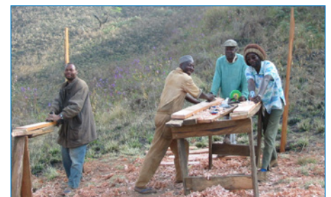
Sawing timber on site
