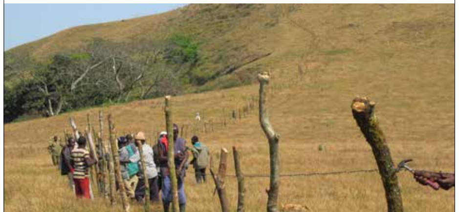
Figure 30. Fences being constructed
