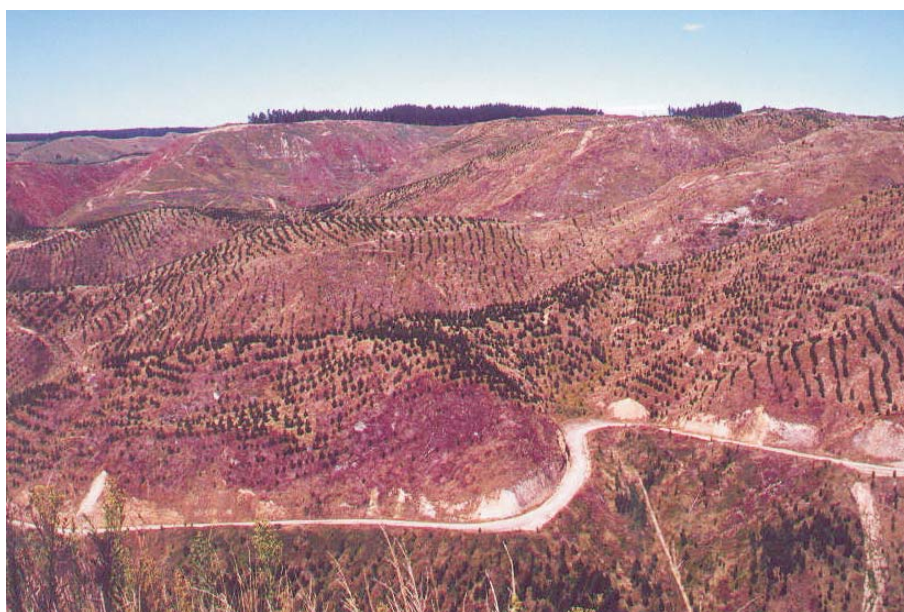
Figure 8. Potential sources of sediment from road cut banks, and sidecast, in the middle reaches of the Pakuratahi catchment.
