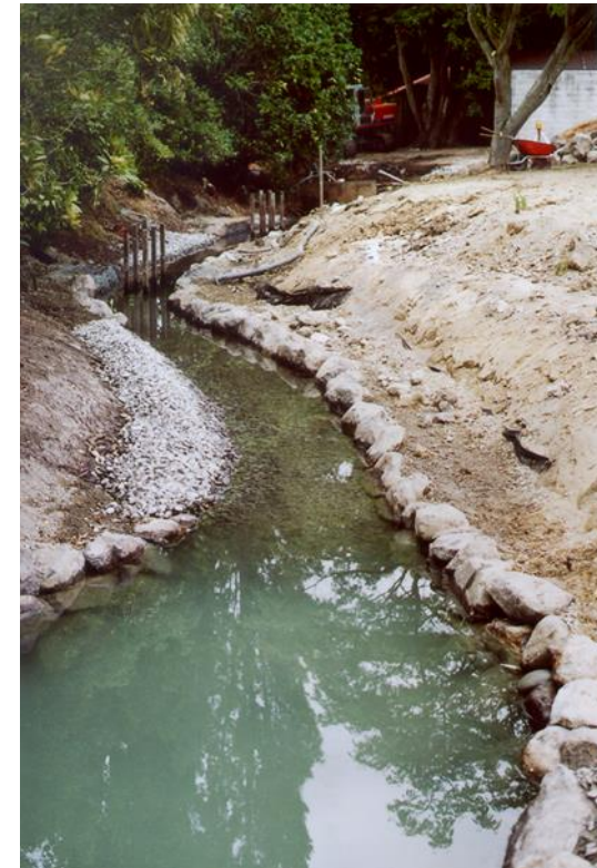
Okeover Stream between Ilam Road and Engineering Road during restoration
