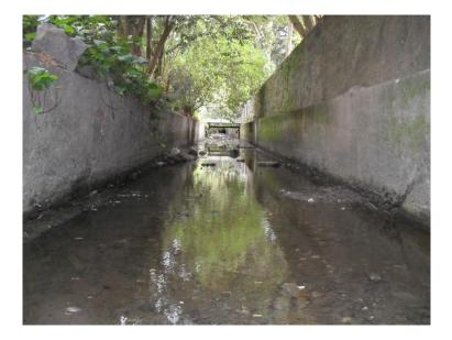
Figure 4: Sumner Stream at Scarborough Beach: Highly modified in box culvert.
