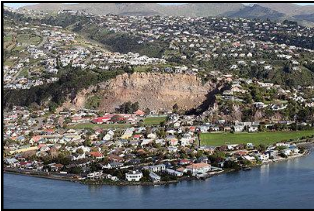
Figure 1: Redcliffs community after the Canterbury Earthquake Sequence
