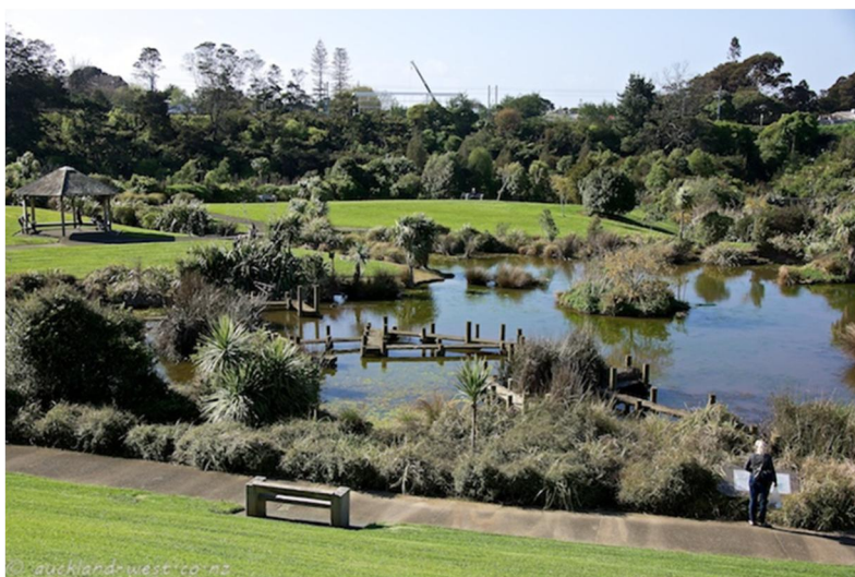
Figure 20. The picture shows a manmade wet pond which was installed in Auckland. This allows water quality and quantity management with regards to stormwater runoff (CCC, 2012).
