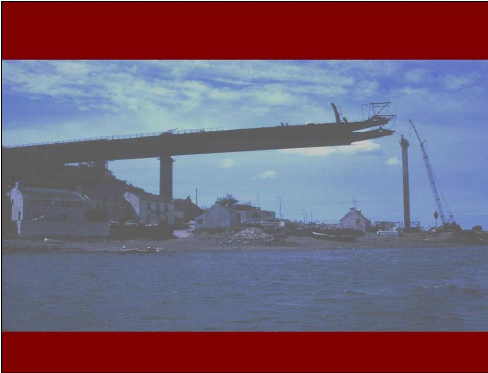
1. On the south side at the equivalent stage the bridge was ready for the last section to be trundled out the next day.
