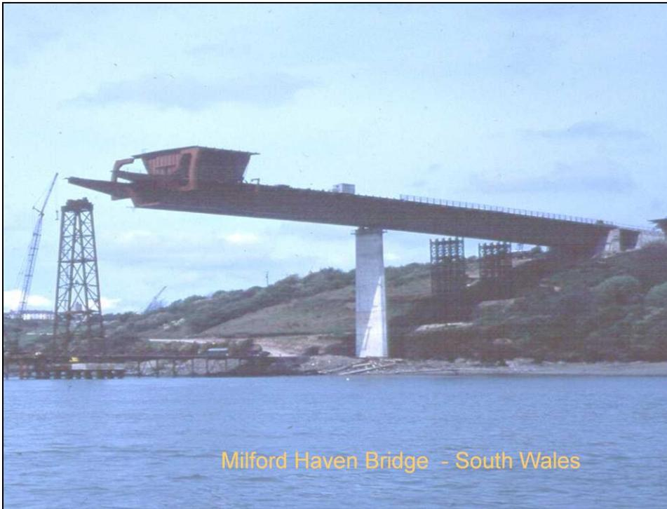
1. One of my first jobs was to assist in the reconstruction of a major steel box girder bridge that collapsed during construction. Milford Haven Bridge.
