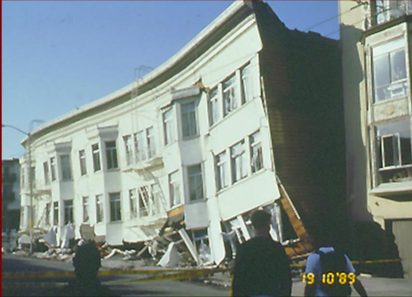
1. Every time there is a major earthquake in a city overseas, we see spectacular and sickening building collapses. More often than not, the prime cause is a critical structural weakness such as a soft storey or plan irregularity. Regular, well detailed buildings, particularly those with shear walls consistently perform well.
