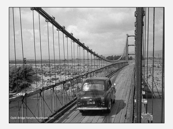
His biggest project was over the Manawatu at Opiki — a main span of 473 feet, with reinforced concrete towers 48 feet high.
