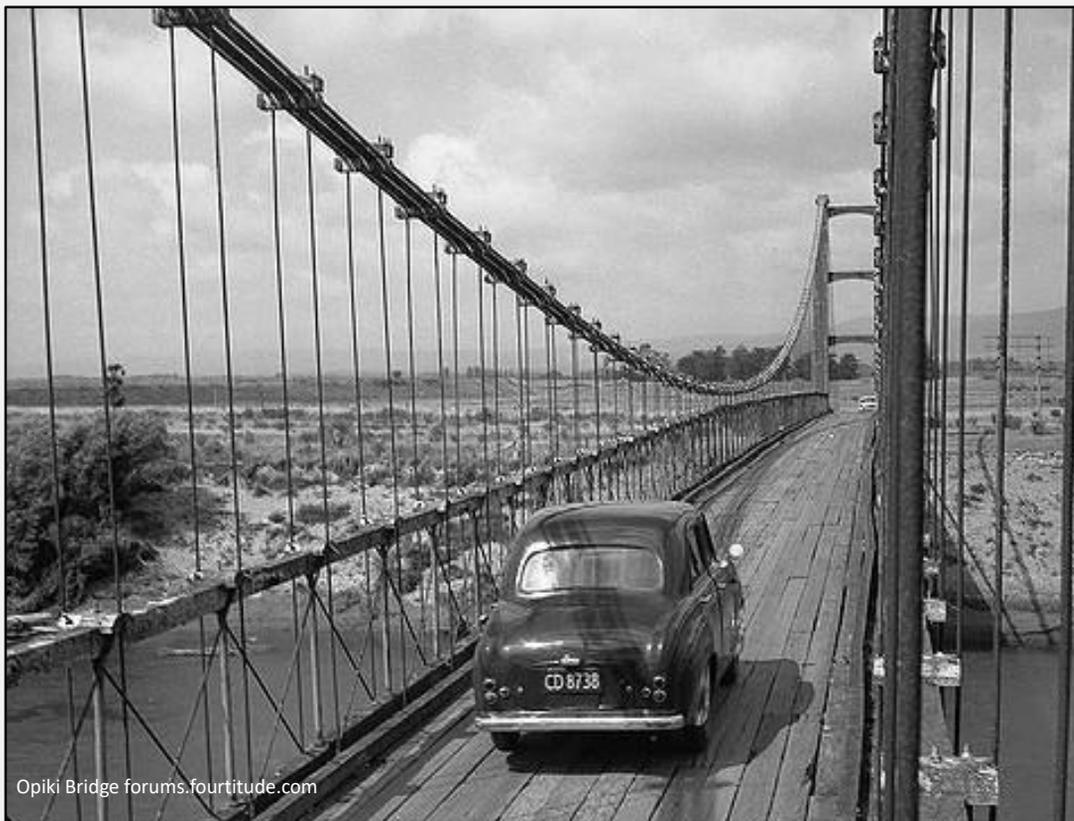
His biggest project was over the Manawatu at Opiki – a main span of 473 feet, with reinforced concrete towers 48 feet high.
