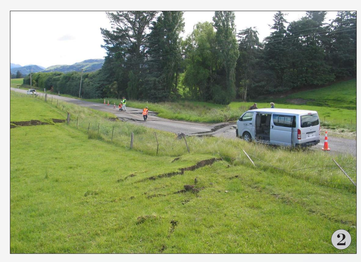
3 Photos depicting the horizontal component of ground displacement (2.2m right lateral) on the Willow Bank strand of the Humps Fault Zone, Inland Kaikoura Road north of Chaffeys Rd.
