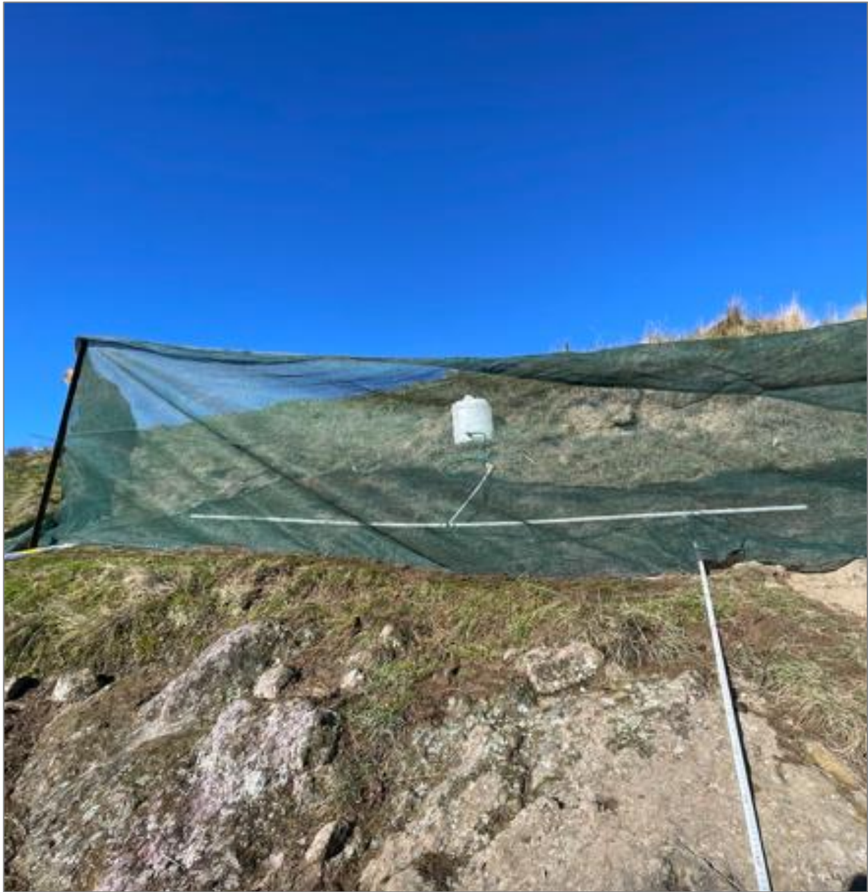
Figure 9: Silt fence attached to the outcrop by 2 posts and inserted into a dug-out trench where possible (Bridgman, 2025).
