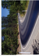
Figure 2. Example of Flushed Pavement. Most common on heavy vehicle traffic routes.
