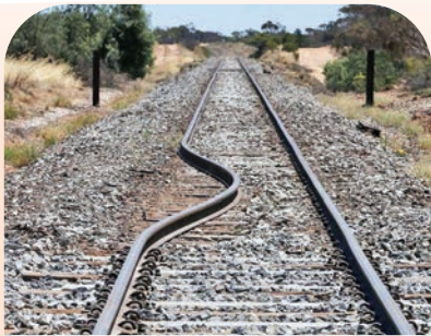
Example of a buckled rail caused by thermal expansion in Victoria, Australia.
