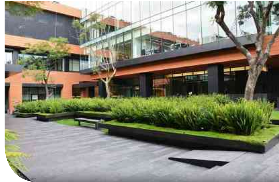
Coyoacán Corporate Campus, Mexico City (DLC Architects)
